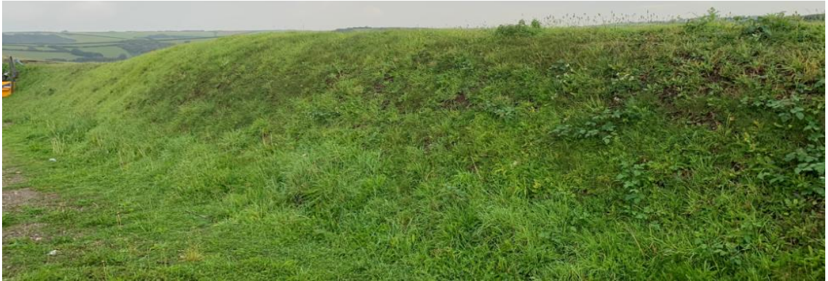
Photo 17: Grass-seeded Soil Storage
