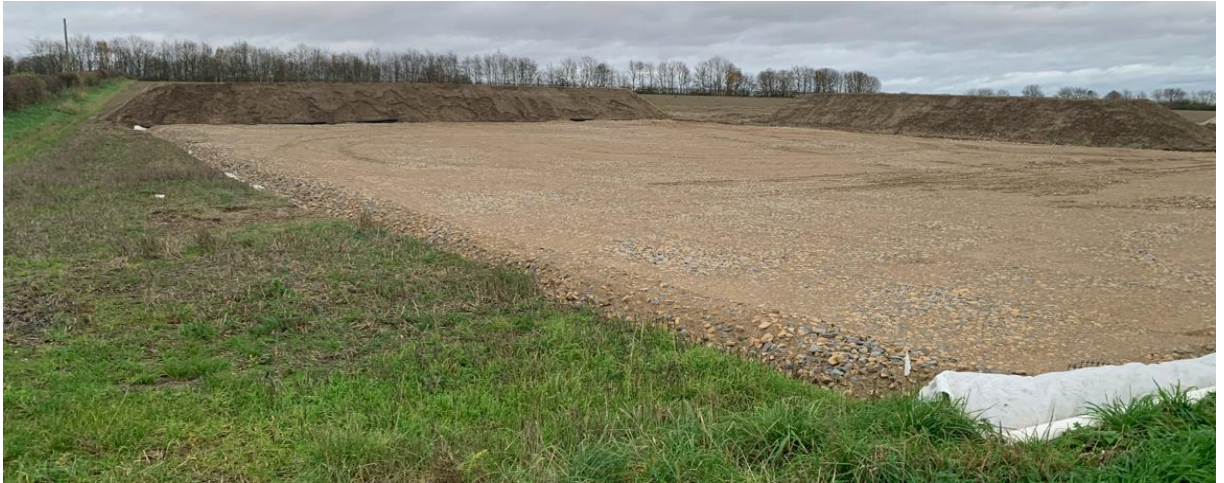
Photo 14: Newly laid Construction Compound (Elsham–Lincoln Pipeline)
